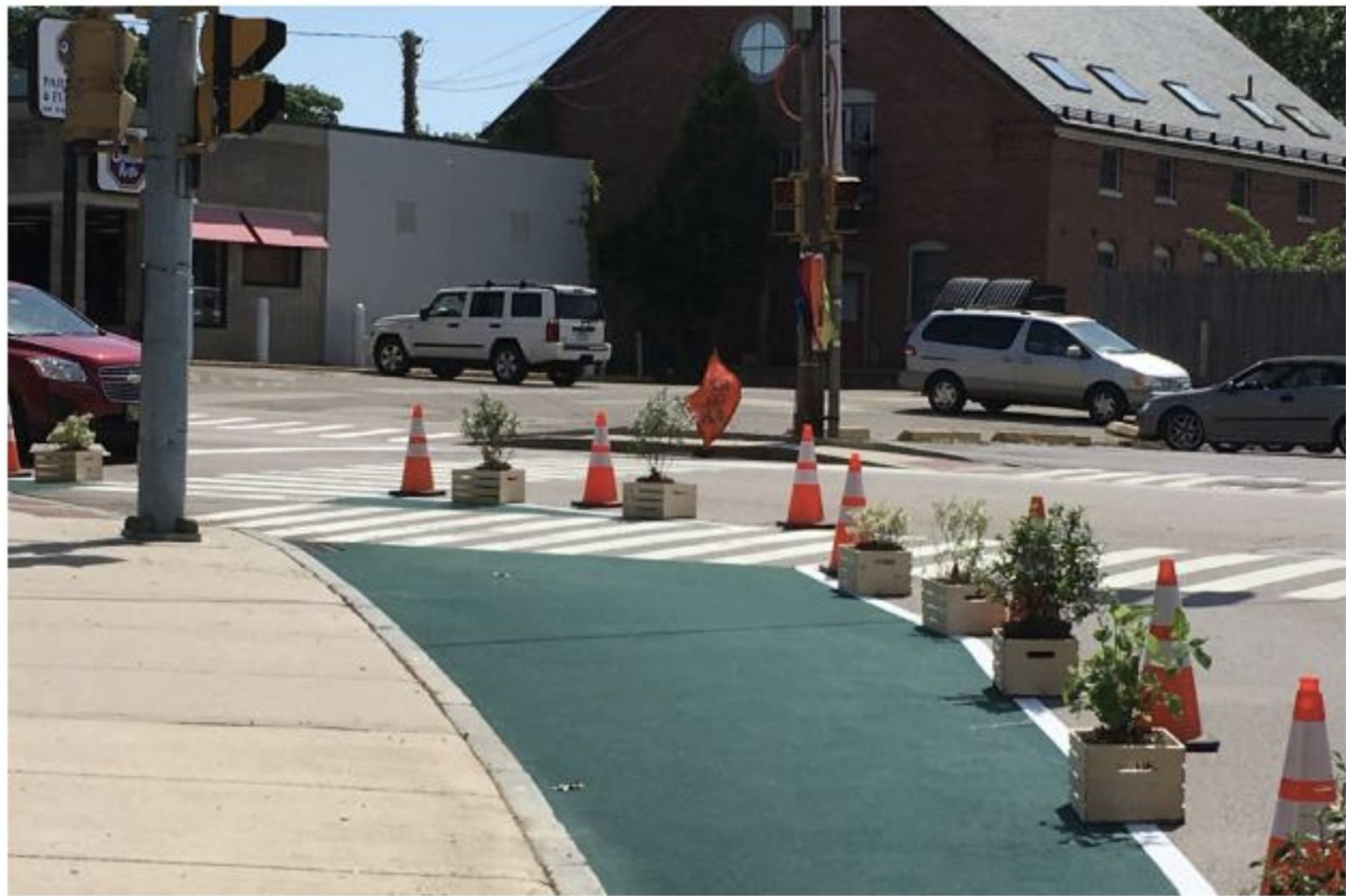
Top: Locally-made wooden crates in Burlington, VT (Street Plans); Bottom: store bought crates used to define the edge of a curb extension in Portsmouth, NH (Street Plans).
